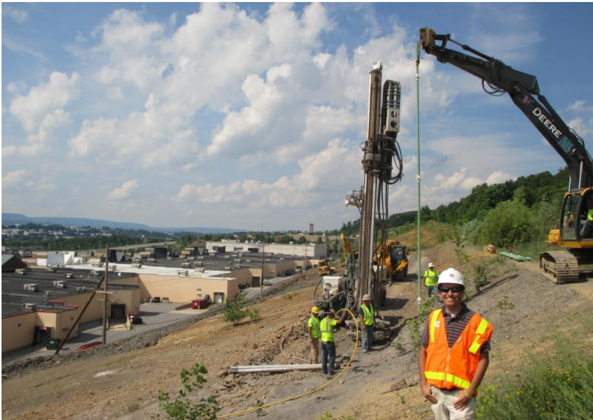
Figure 8. Installation of First Micropile at the Site
