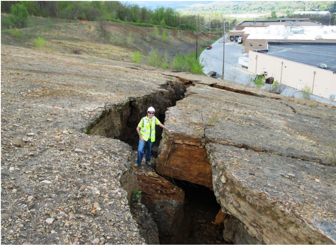
Figure 5. Tension Crack at top of the Rockslide
