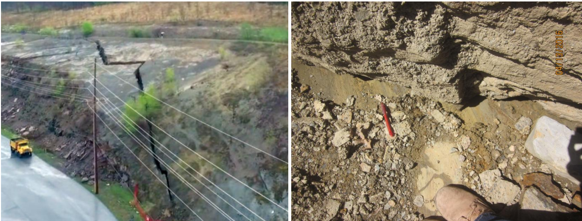
Figure 6. Overview of the Rockslide and Closer View of the Failure Plane.
