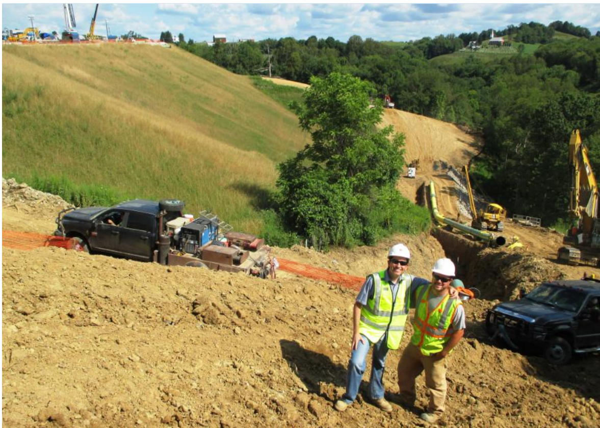
Figure 4. Pipeline Installation After Construction of the 75 Drilled Shafts
