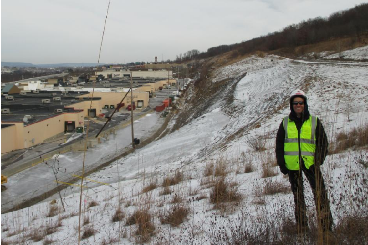
Figure 9. Installation of First Micropile at the Site
