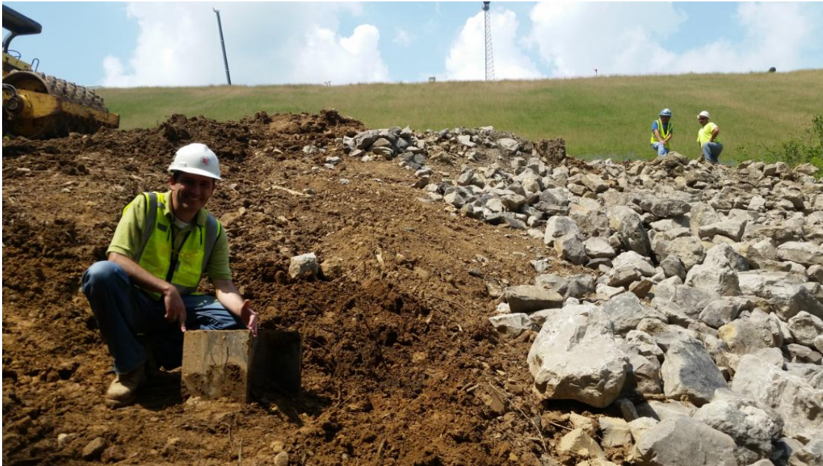
Figure 3. Terminated Drilled Shaft/Steel Section after Construction
