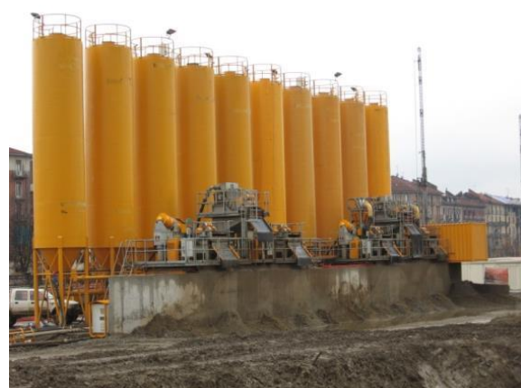
Figure 8. Bentonite storage in tanks (left); Desanding plant and bentonite storage in silos (right)
