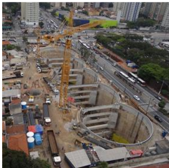
Figure 26. Shafts after final excavation
