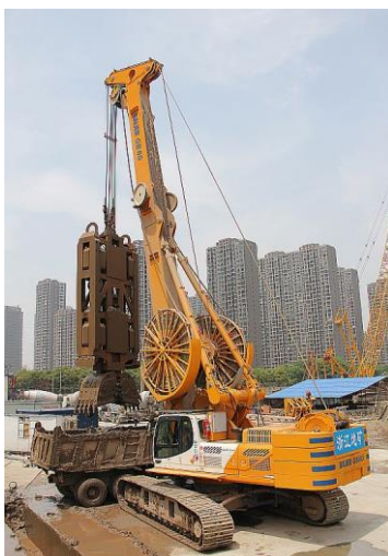
Figure 12. Loading process for grab (left), Slurry circuit for trench cutter (right)
