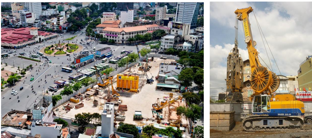
Figure 21. Job site overview (left), GB 46 Grab at work (right)
